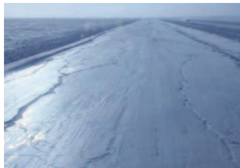
Normal longitudinal cracking caused by buoyancy of the thickened ice over the 20-metre-wide travel lane
