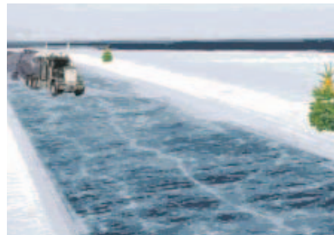
Marked pine trees cut and placed as reference markers along an ice road
