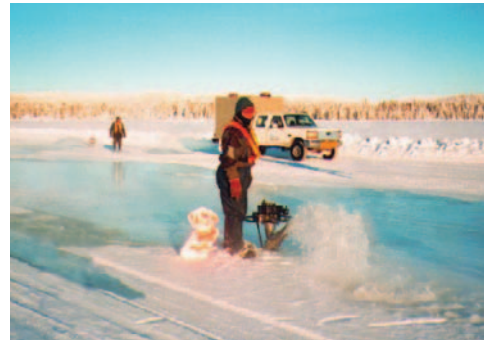
Flooding crew repairing an ice road
